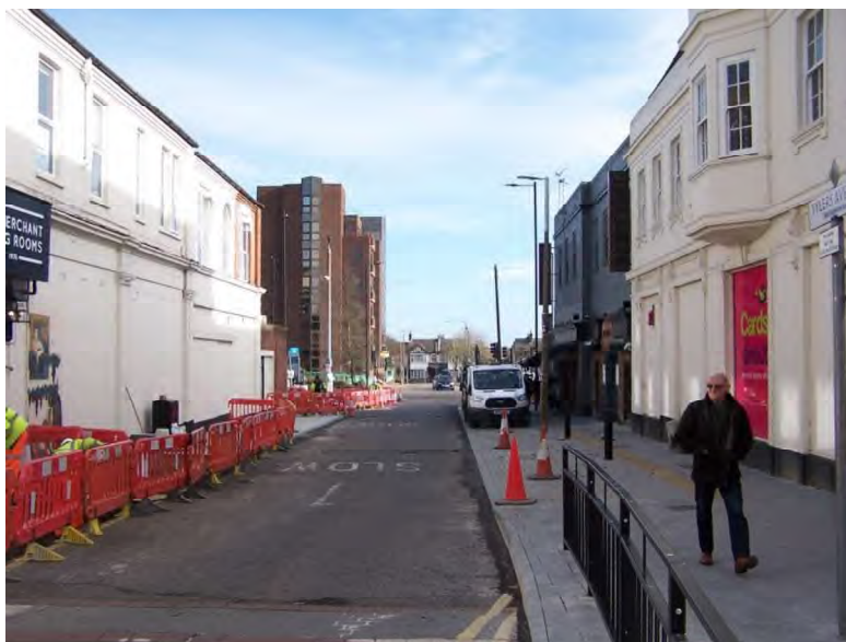
Figure 10: View along Tylers Avenue from the impact point
