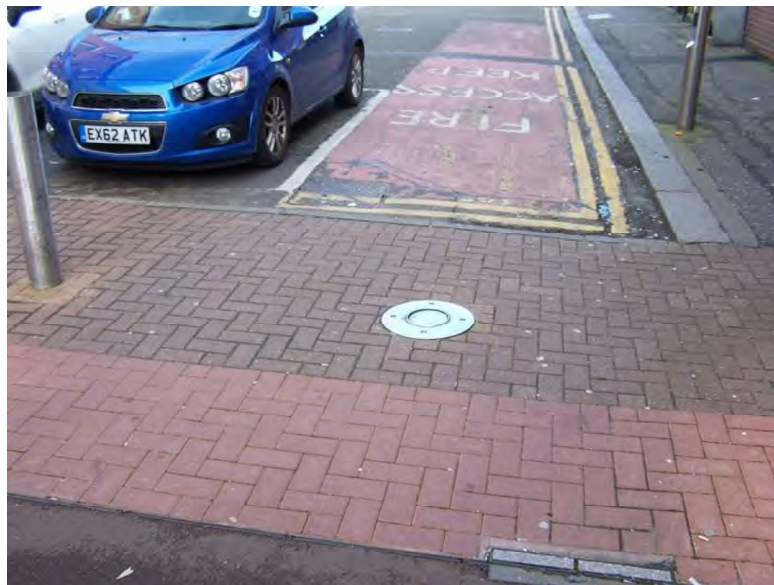
Figure 9: Route 7 impact point retractable bollard
