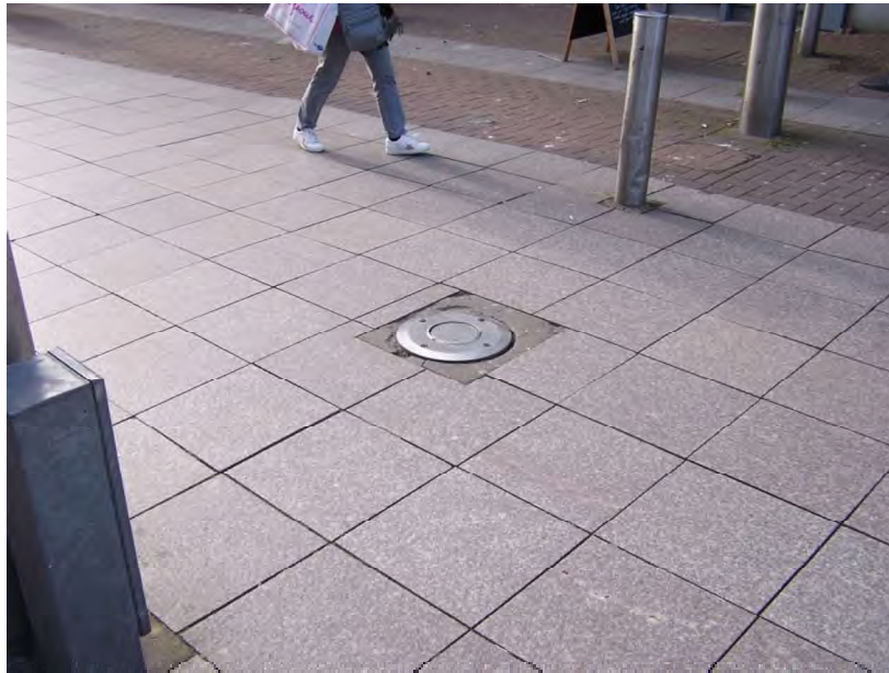
Figure 17: Approach route 10 impact point rising bollard down allowing vehicle access.
